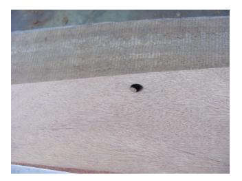
The goal is to clean out the hole with a drill bit and then plug the hole with one or more bungs. The problem is that sometimes the hole is at a significantly oblique angel, which makes starting the drill difficult. In that case I make a drill guide out of scrap wood, clamp the guide to the plank the drill.
